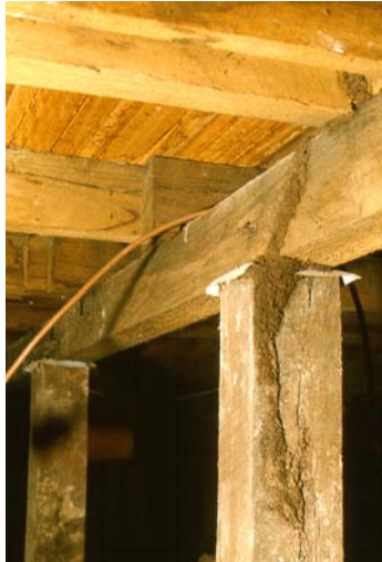
FIGURE D1 TERMITES BRIDGING TERMITE CAP BY MEANS OF A SHELTER TUBE
